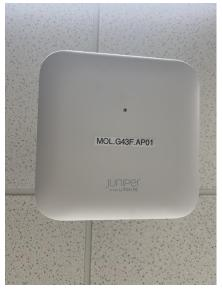
NOTE: for APs that are in enclosures, a label must also be added in a clearly visible location on the enclosure itself as shown on this example.
